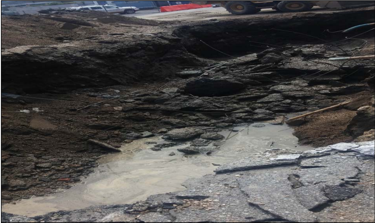
View of removal of bottom slab (looking south)
