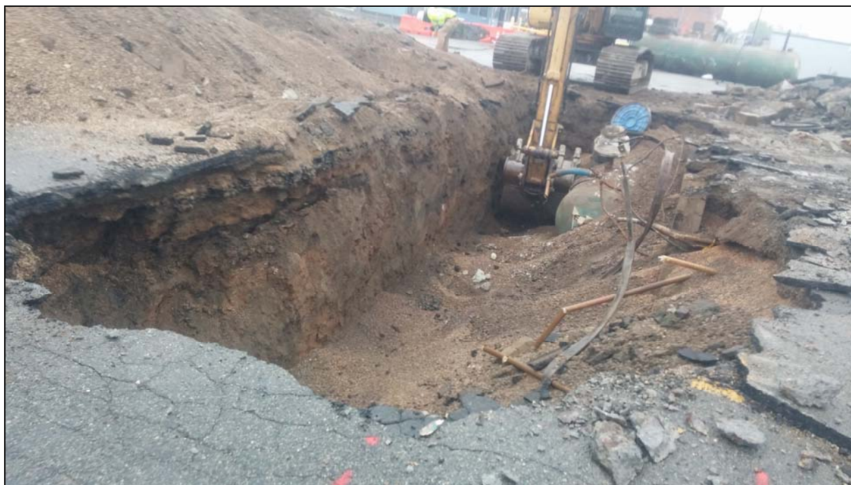
View of 1,000-gallon diesel UST in Excavation (looking south)
