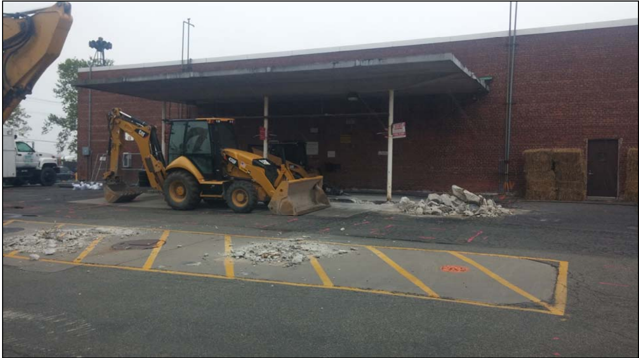
View of former tank mat before underground storage tank (UST) removal (looking west)
