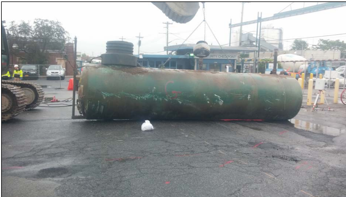
View of former 4,000-gallon gasoline UST (looking east)
