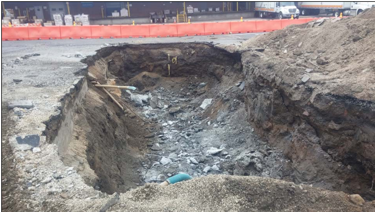
View of broken up concrete bottom slab (looking north)
