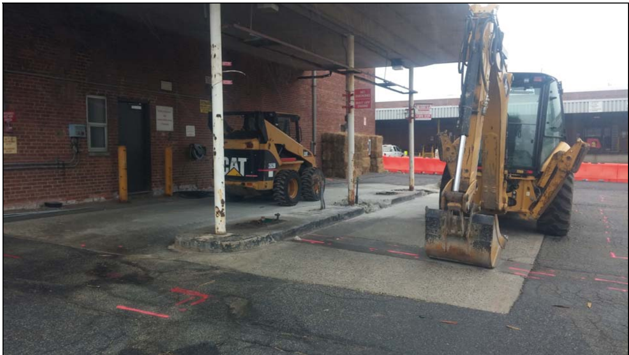
View of former dispenser area (looking north)
