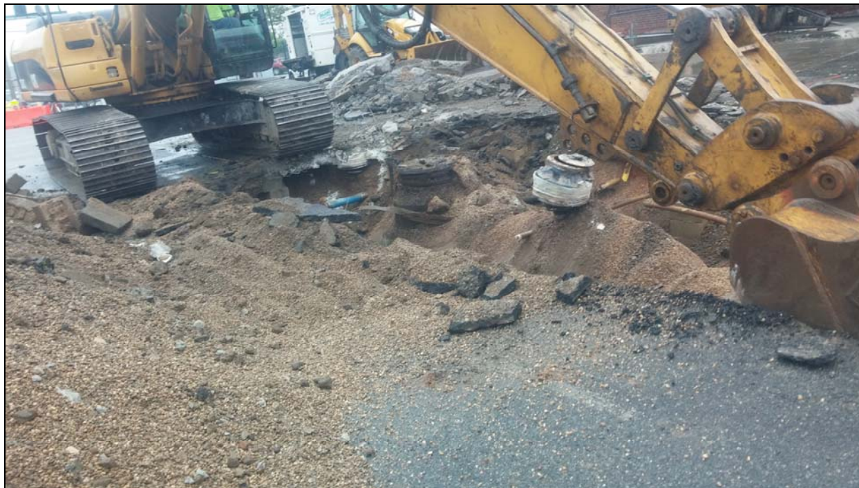
View of 4,000-gallon gasoline UST in Excavation (looking southwest)
