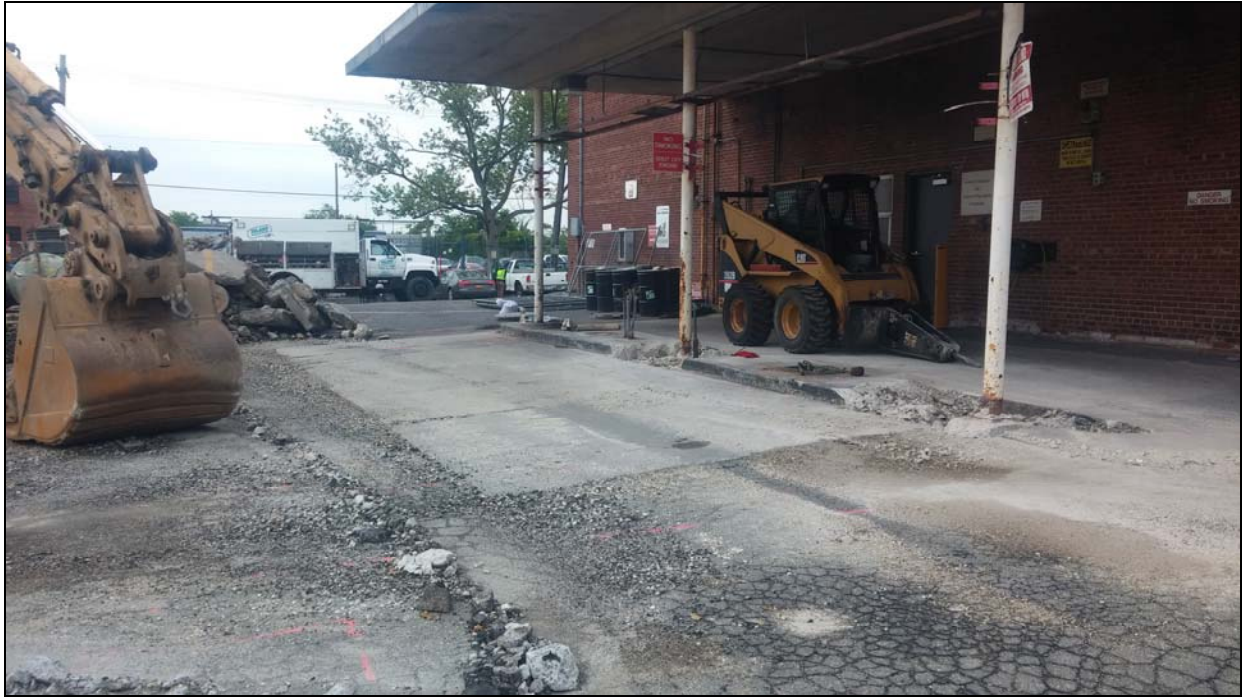
View of former dispenser area (looking south)
