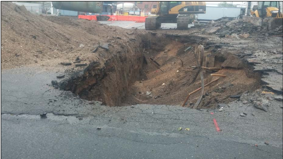
View of open excavation (looking south)
