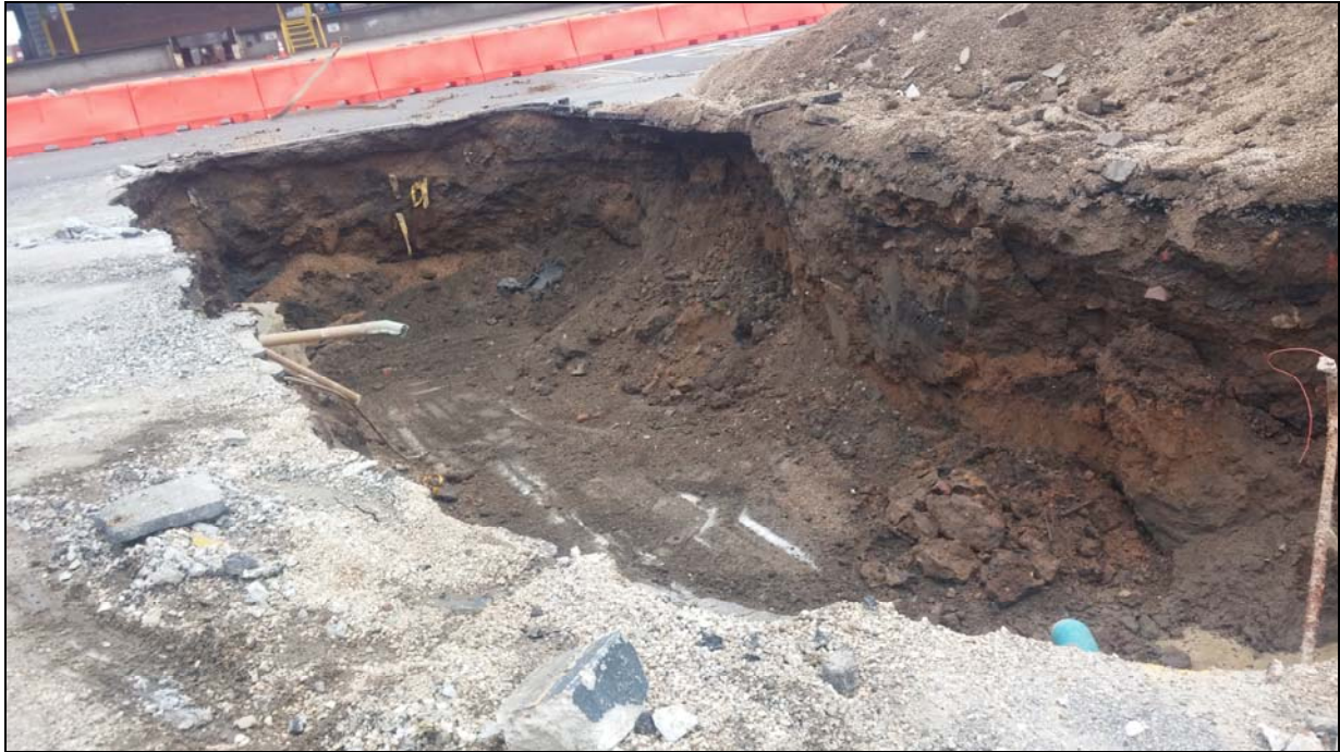
View of concrete bottom slab (looking north)
