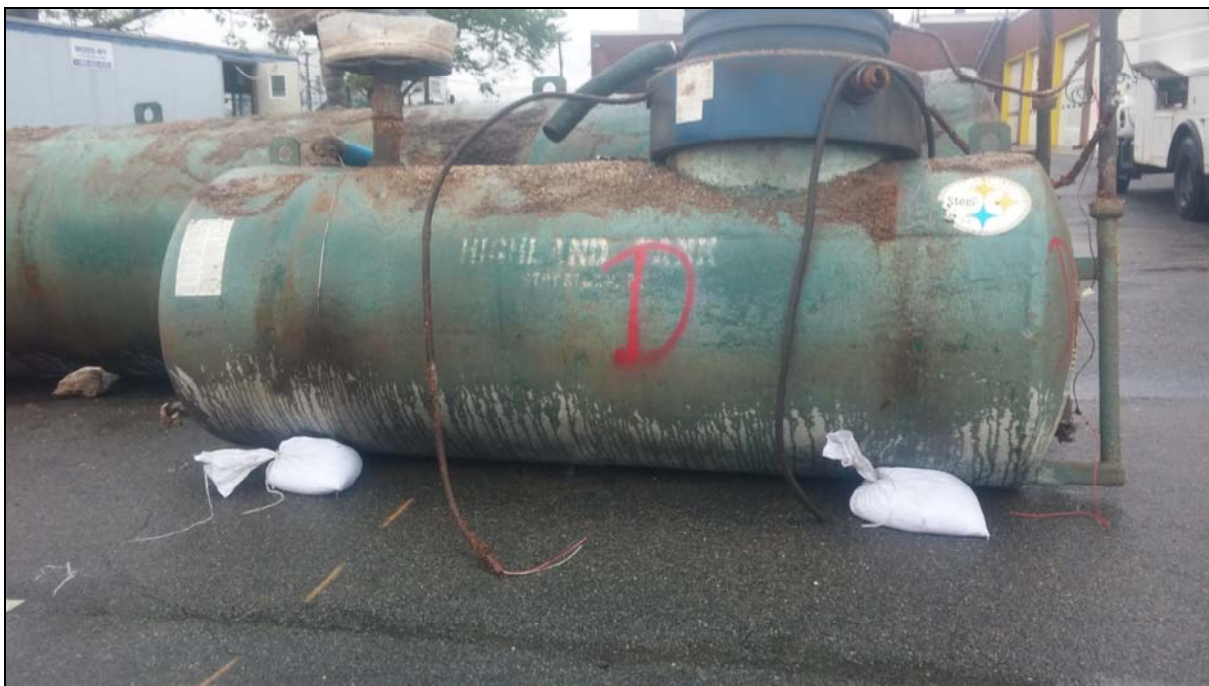
View of former 1,000-gallon diesel UST (looking west)
