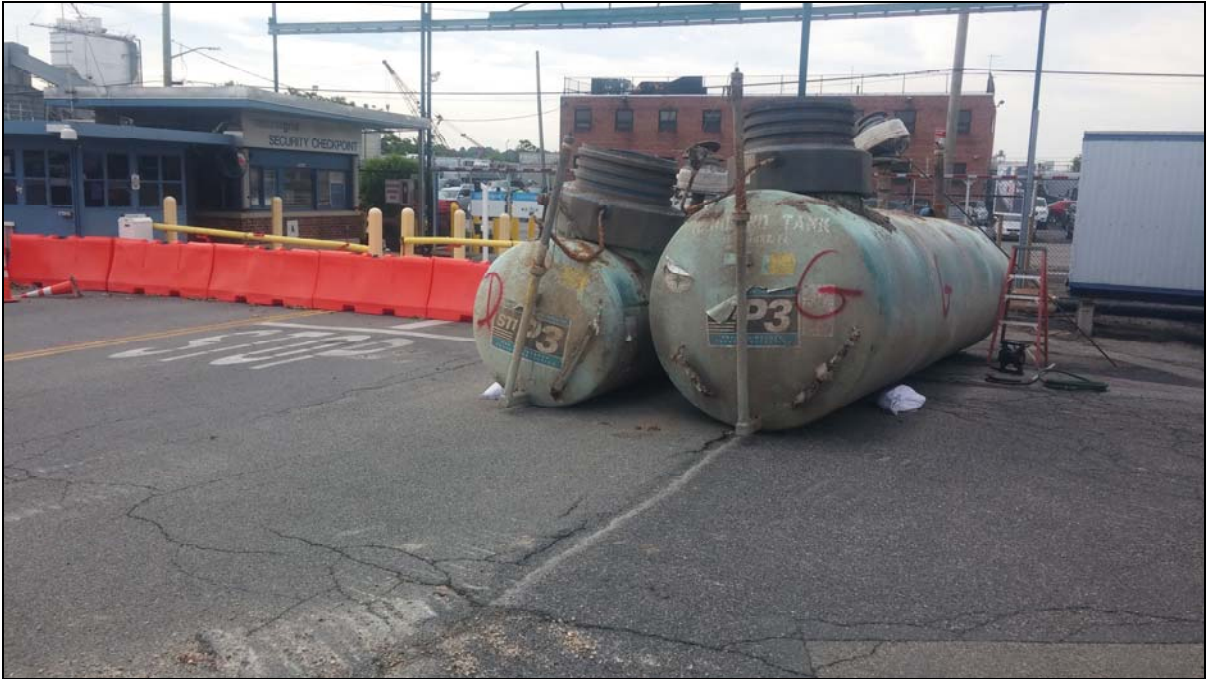
View of former 4,000-gallon gasoline and 1,000-gallon diesel USTs (looking south)
