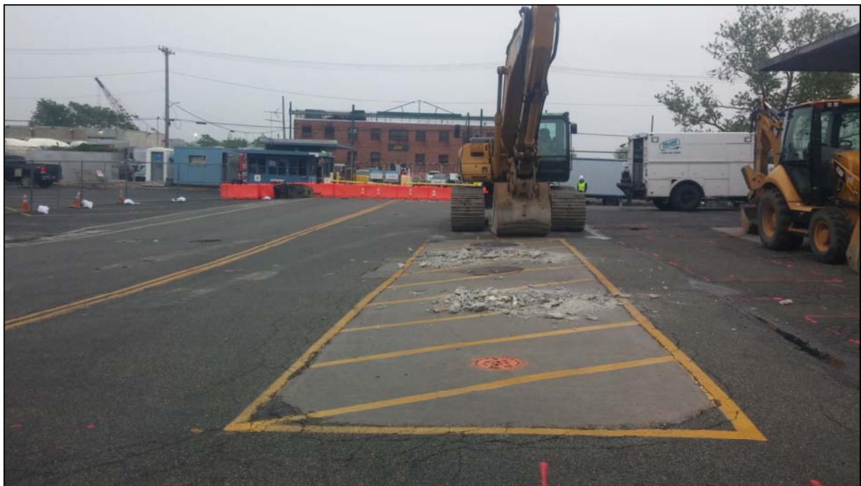
View of former tank mat before UST removal (looking south)
